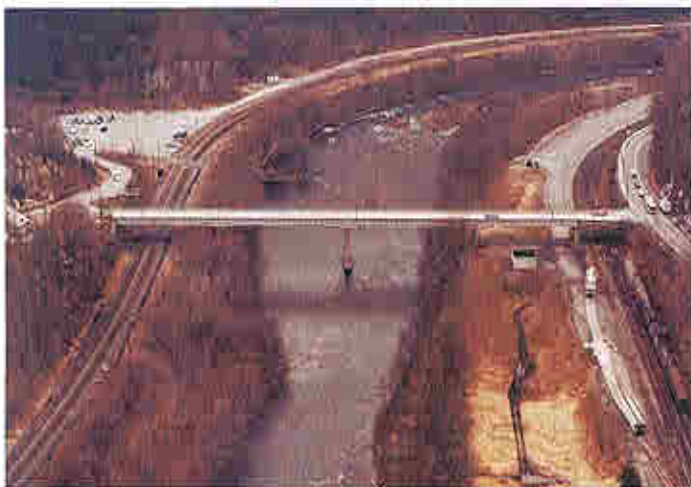
The existing Jim Thorpe Bridge.
